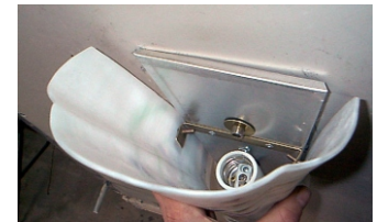
Placing back plate reflector over mounting stud
