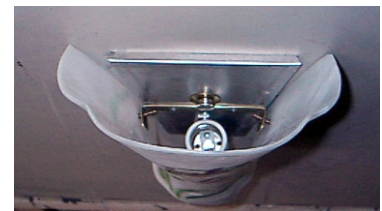
Sconce mounted snug to wall with knurled nut.
