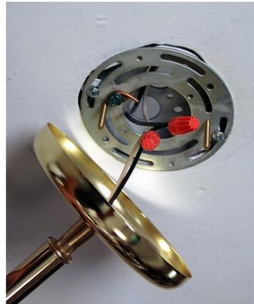
Fixture bracket attached to electrical box. Note the two bolts extending from the bracket. Canopy with drop tube attached is on the left and the fixture wires are connected to the supply wires by the wire nuts. Be sure to use the toothed locknut under the hex nut attaching the canopy to the drop tube assembly.
