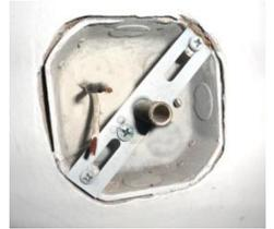
Wall box with fixture bracket and mounting stud installed
