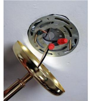
Attaching drop tube assembly to the electrical box. Note the two bolts extending from the bracket. Canopy with drop tube attached is on the left and the fixture wires are connected to the supply wires by the wire nuts. Be sure to use the toothed locknut. Note also that the swivel lies right below the canopy.
