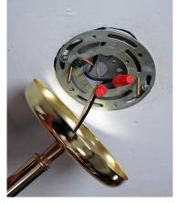
Fixture bracket attached to electrical box. Note the two bolts extending from the bracket. Canopy with drop tube attached is on the left and the fixture wires are connected to the supply wires by the wire nuts. Be sure to use the toothed locknut under the hex nut attaching the canopy to the drop tube assembly.
